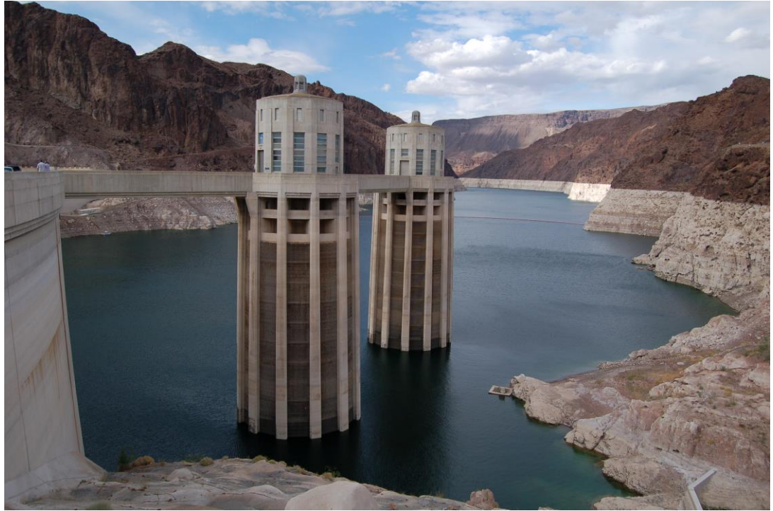
Figure 1. Lake Mead water level as of 2010. The white “bathtub” ring reflects exposed rock that was previously underwater. The ring shown here is approximately 130 feet (40 m) (©Photo by Lynn F. Fenstermaker, used with permission.)
